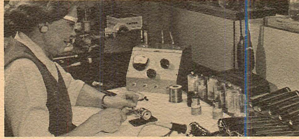
Soldering microphone pressure unit assembly into microphone chassis.
